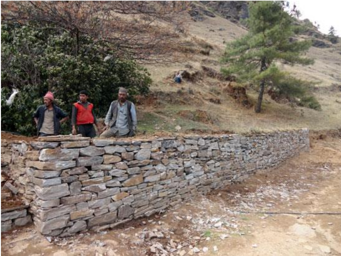
Figure 12 local Fence work at medical center
