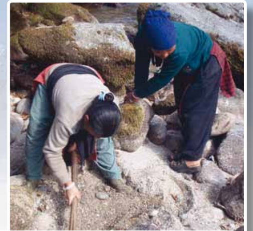
Local women collecting sand from the river for the 2010 work group
