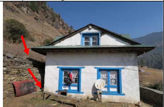
Staff quarters, peak & crack repairs Arrows indicate new drain locations
