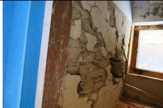
Toilet block internal walls need repair
