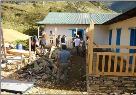
Work group building a verandah
